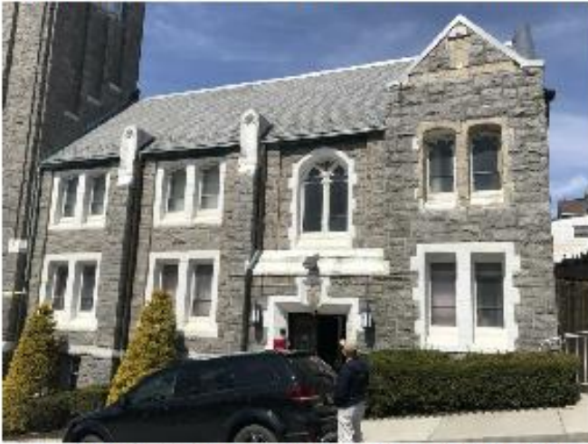
1) UPPER END OF MAUCH CHUNK SIDE BELOW THE TOWER
