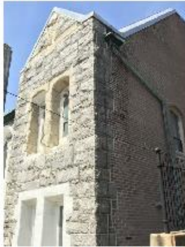
2) NO WORK TO THE BRICK RETURN DOWN THE ALLEY
