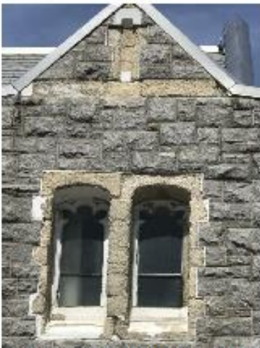
3) UPPER END OF MAUCH CHUNK SIDE BELOW THE TOWER
