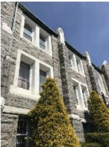
5) UPPER END OF MAUCH CHUNK SIDE BELOW THE TOWER
