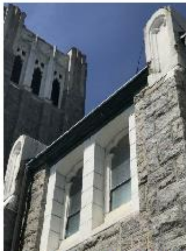
4) UPPER END OF MAUCH CHUNK SIDE BELOW THE TOWER
