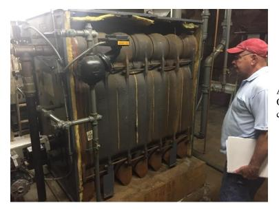
AFTER - The boiler was disassembled and the sections cleaned. One section had to be replaced. All O-rings were replaced. Total cost: \$13,000
